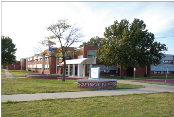
ESCUELA SECUNDARIA SOUTHEAST 5401 S. SHIELDS OKLAHOMA CITY, OK 73129 587-9600
